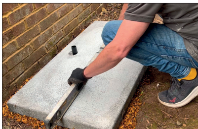
STEP 5 - Ensure that slab is level.
