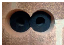
3. INSERT THE PVC SLEEVE INSULATION, RECESS IT TO ALLOW FOR THE ELBOW TO BE LOCATED.
