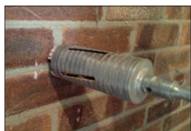
1. SELECT A 65MM CORE DRILL.
