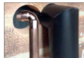
4. FIT THE ELBOW OVER THE COPPER PIPES.
