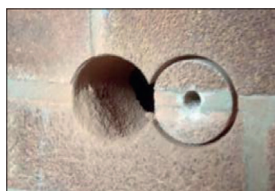
2. DRILL TWO 65MM HOLES NEXT TO EACH OTHER.
