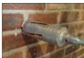
1. SELECT A 65MM CORE DRILL.
