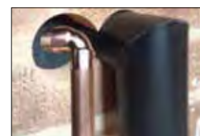
4. FIT THE ELBOW OVER THE COPPER PIPES.
